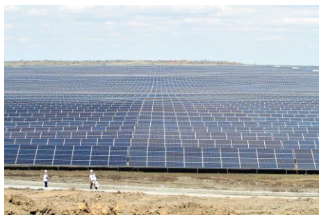
Nikopol Solar Park (DTEK), Dnipropetrovsk Oblast Capacity – 246 MW Consists of 750 000 operational units
